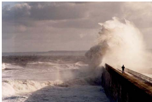
Fig. 1.1: Overtopping on sea wall
