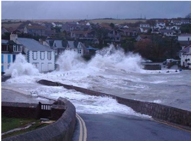
Fig. 1.2: Flooding caused by overtopping
