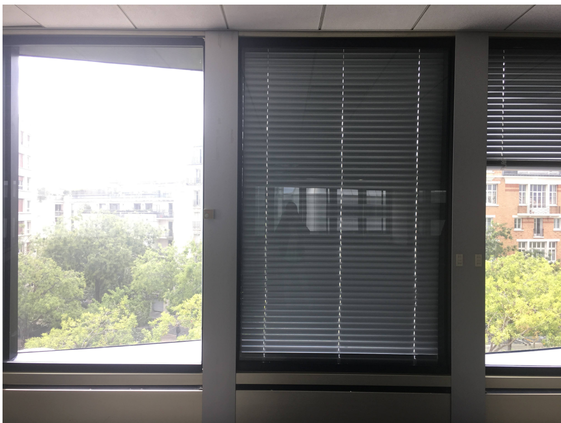
Figure 3.2: Inside view of the double skin façade
