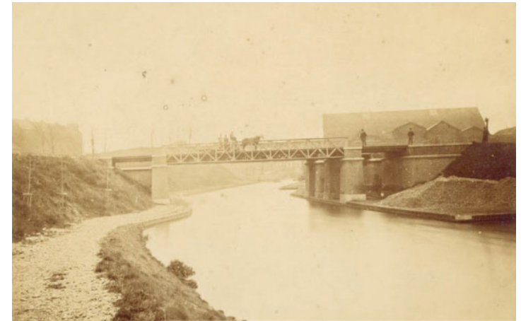
Photo of the bridge to Sappi, seen from the north, date unknown (source: srhclimborg).
