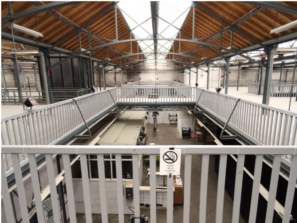
First floor. Vides creating look through into the building and brings light to the ground floor.
