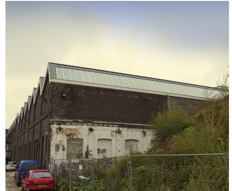
North facade warehouse, photograph.
