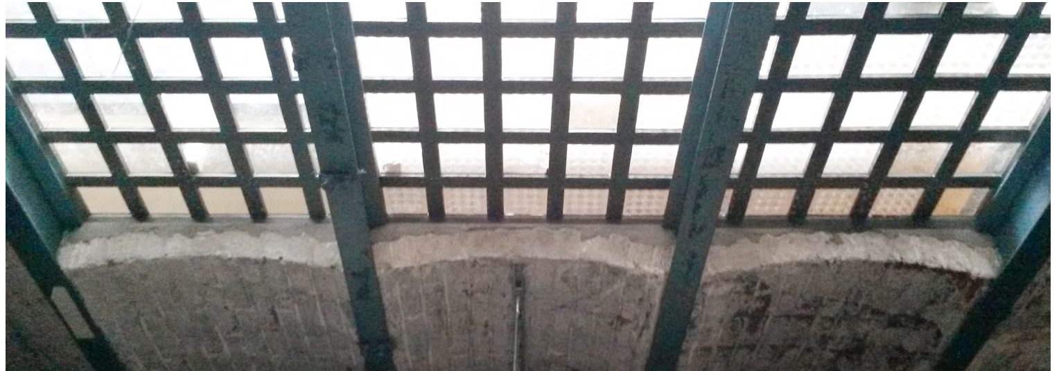
Photograph of the ground floor, taken from the basement.
