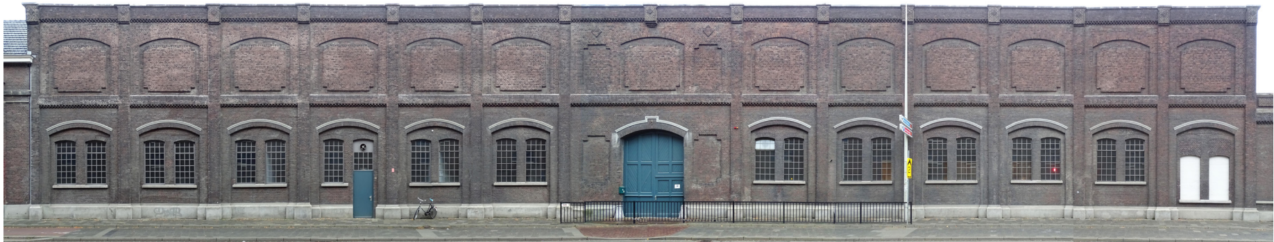
West facade warehouse, photograph.
