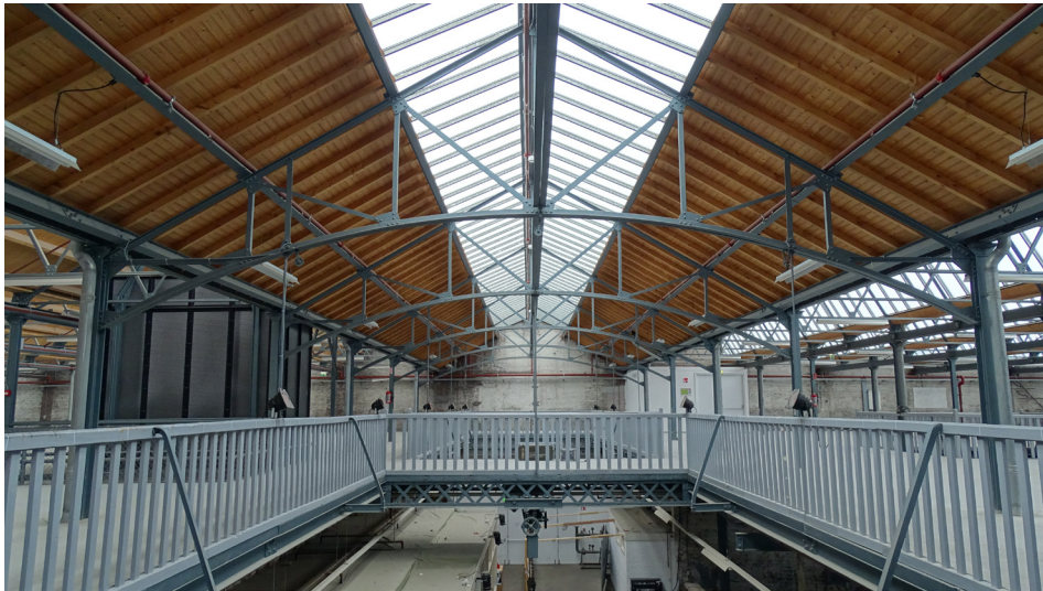
Photograph of gable roof structure above the main street.
