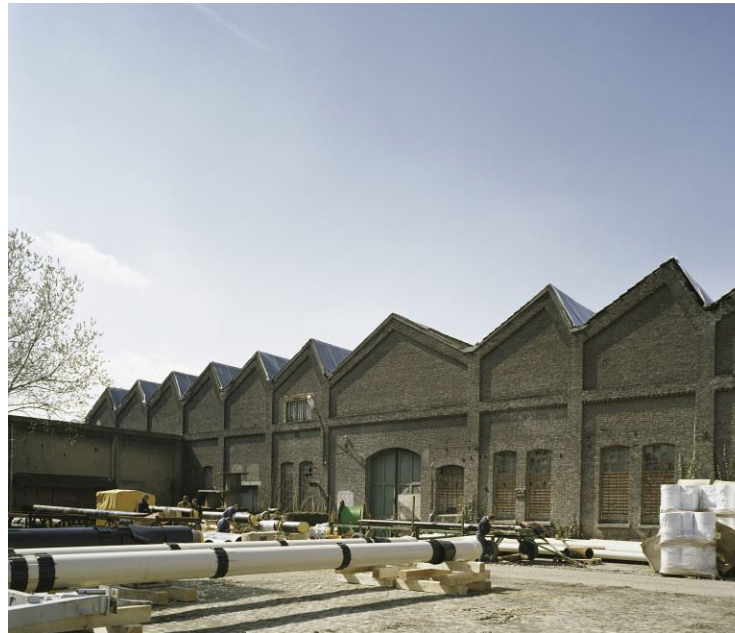
East facade warehouse, photograph from the inner court (2006, RCE).
