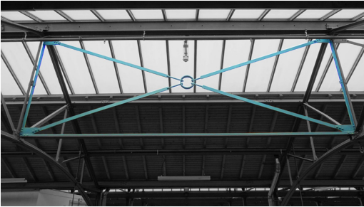
Stability shores in the roof construction.
