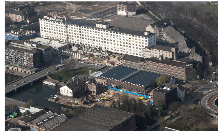
Aerial view on the area in 2015. A new bridge has appeared and a lot of buildings have been demolished (source: Blackboard TU Delft ).
