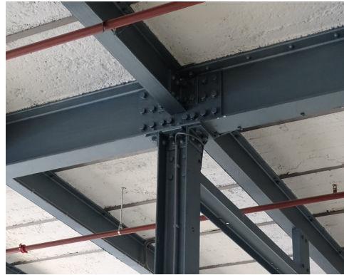
Close up of column, beam and floor connection.
