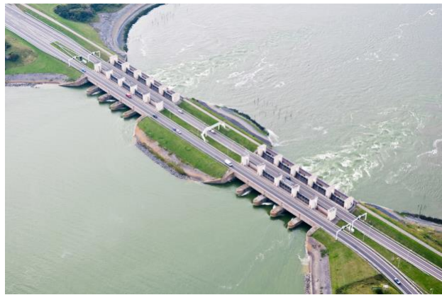
Figure 36 Photograph of the outlet sluices of Kornwerderzand. Source: Houdt (2011)
