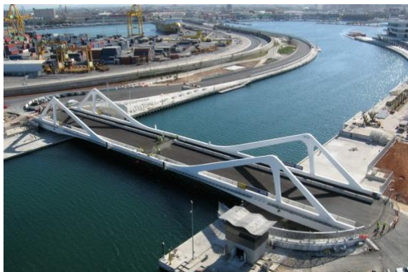
Figure 49 Valencia Port Swing Bridge opened for traffic (MC2 Estudio De Ingenieria , 2017)
