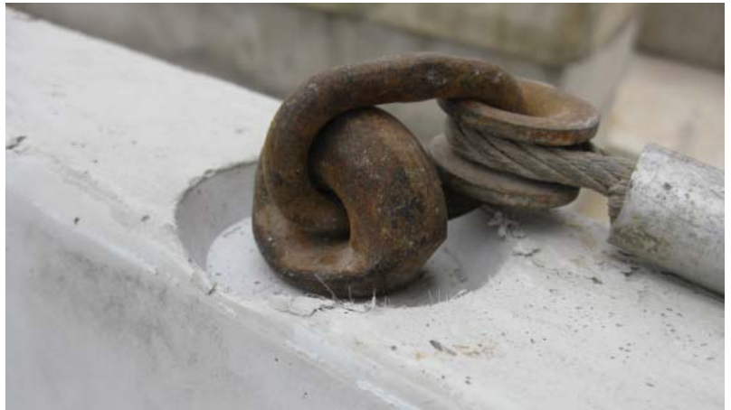
fig.8.8 embedded anchor in the thickness (60mm) of the panel
