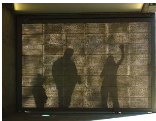
fig.2.2 translucent concrete panels produced by Litracon www.litracon.hu
