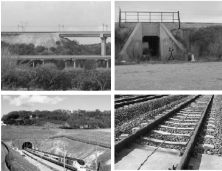
Figure 1.1: Most common types of railway transitions zones [28].
