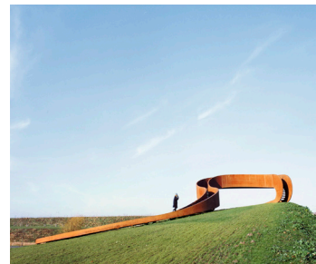
Example of an merging interpretation: The Elastic Perspective, by NEXT Architects, Barendrecht.
