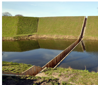
Example of an merging interpretation: Moses Bridge, by RO&AD Architects Halsteren.
