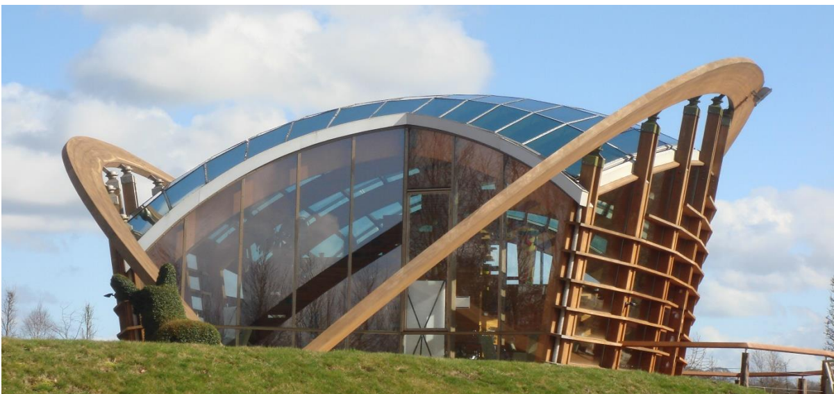
Figure 4: Iroko glued laminated structure.
