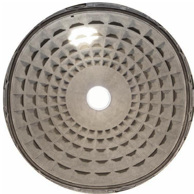
Figure 2.18. Interior of the Pantheon dome, seen from beneath. The concrete for the coffered dome was laid on moulds, mounted on temporary scaffolding. (Kabel, 2008)
