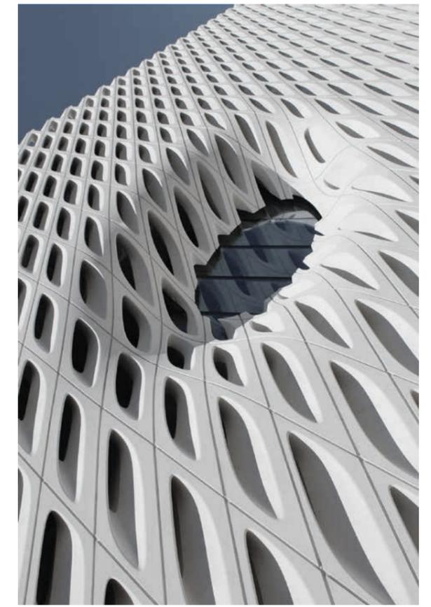
Figure 2.22. Non-load bearing GFRC facade panels, Broad Museum, Los Angeles by Diller Scofidio + Renfro (WillisConstruction, 2015)
