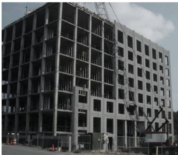
Figure 2.9. Fixing the non-load bearing concrete facade panel under construction, Proximity Hotel (Pearce & Ahn, 2013)
