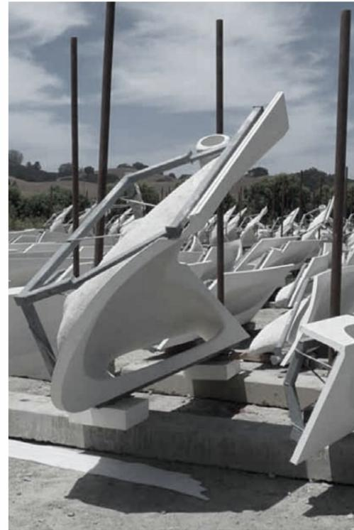
Figure 2.71. Drying of GFRC casted facade panels (Gensler, 2015).
