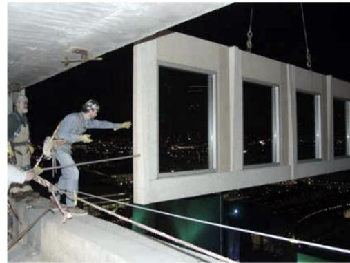
Figure 2.66. Erection of precast concrete facade wall with pre-installed windows using tower crane (Boswell et al., 2016).
