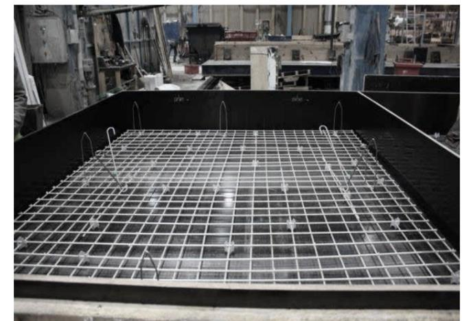
Figure 2.25. Glass fibre woven textile reinforcement for concrete casting (Malaga et al., 2012)
