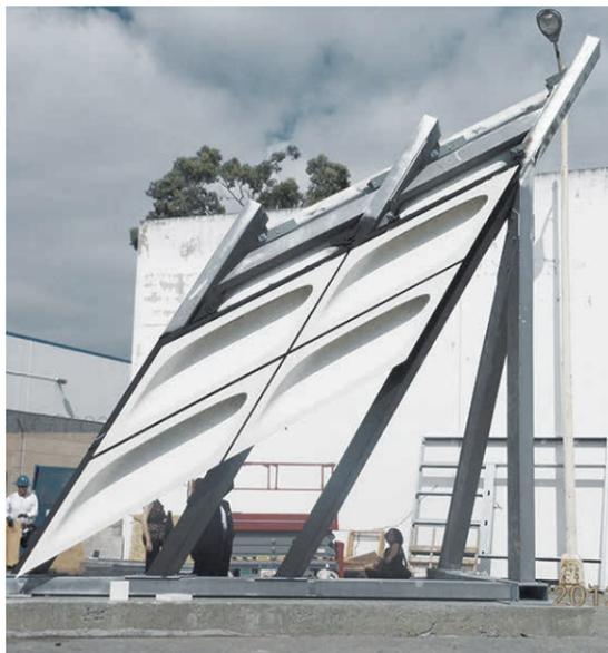
Figure 2.72. Spray up casted panels fixed to one module of steel member support (Lubell, 2014).
