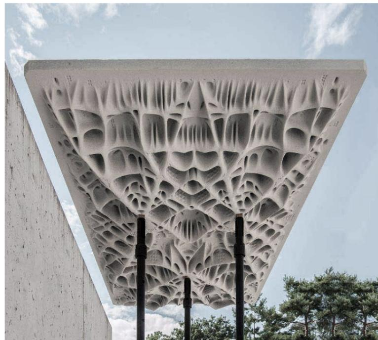
Figure 2.60. Prototype A: Topology optimisation of a concrete slab with three point support (Jipa et al., 2016).
