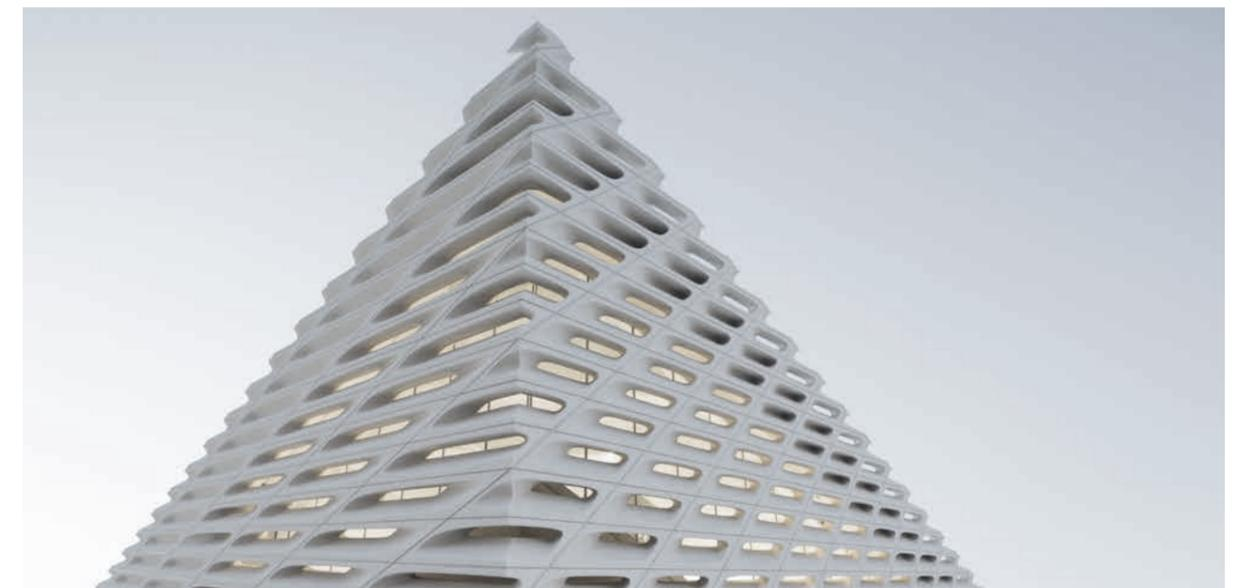
Figure 2.69. The Veil facade comprised of 2500 GFRC panels with window opening in each of them. (Bianchini, 2016).
