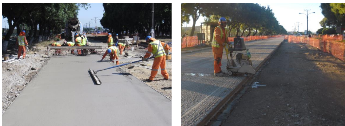
Fig. 5.4.4 Paving with formwork (left) and saw-cutting the transverse joints (right) of the Chilean JPCP.
