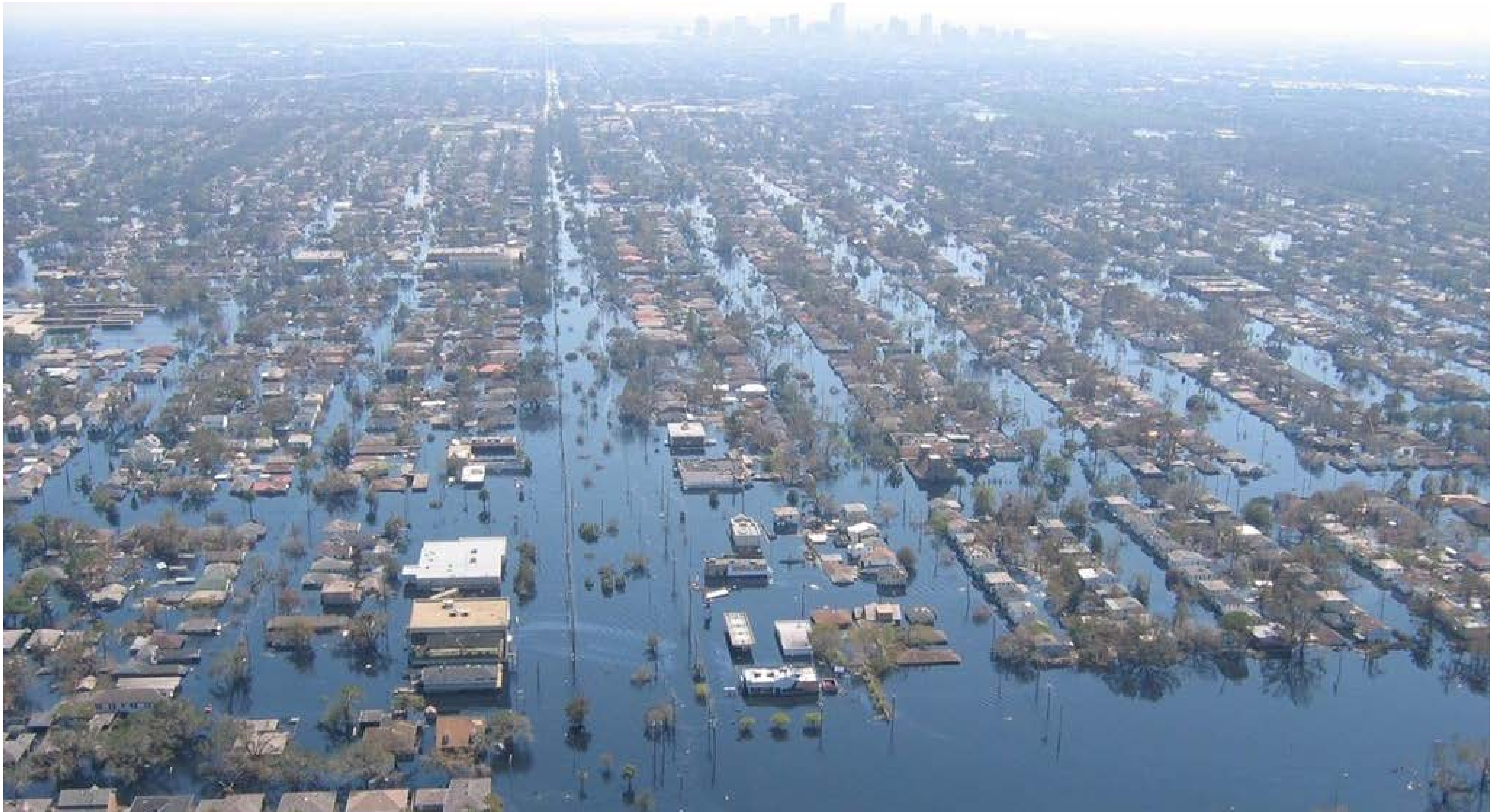
Impact of hurricane Katrina. source: architect
