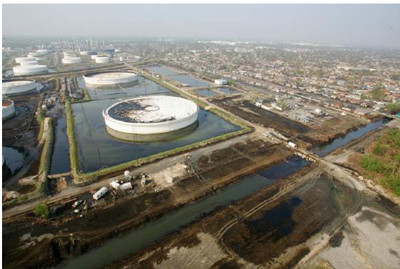
Figure 5.1. A massive oil spill that threatens this town in St. Bernard Parish resulted when an oil tank was forced from its foundation by Hurricane Katrina's massive storm surge. (Courtesy of Bob McMillan/ FEMA)
