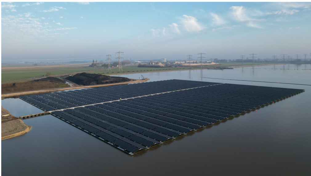
Figure 2.1: Aerial photograph of a floating solar installation on an inland water body [14].
