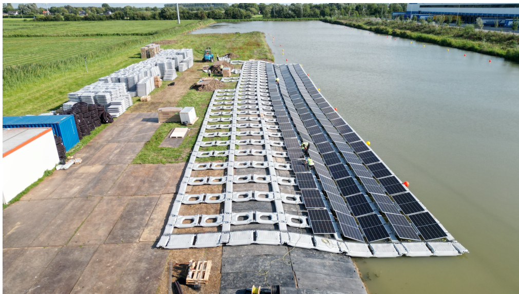
Figure 2.3: Floating solar installation during assembly, showing the modular HDPE floater structure [14].
