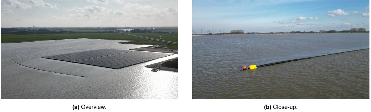
Figure 2.11: HDPE pipe wave barrier at a floating solar installation. (a) Overview showing the pipe as the dark floating line encircling the FPV system. (b) Close-up of the pipe and mooring connection at the water surface [14].
