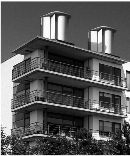
Aromine rooftop wind turbine, applied to a housing building.
