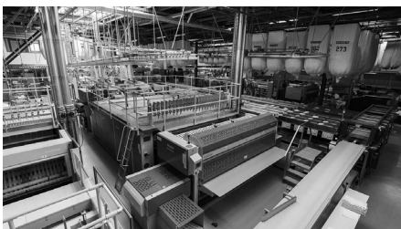
Jensen semiautomated laundry facility in Meuse, Belgium.
