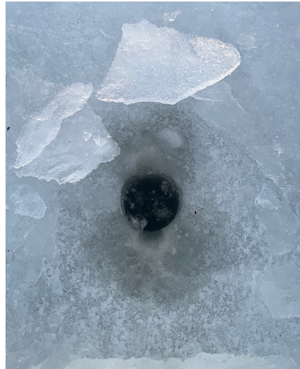
(b) Photograph of hole 4 showing upward spalling observed in both test directions.
