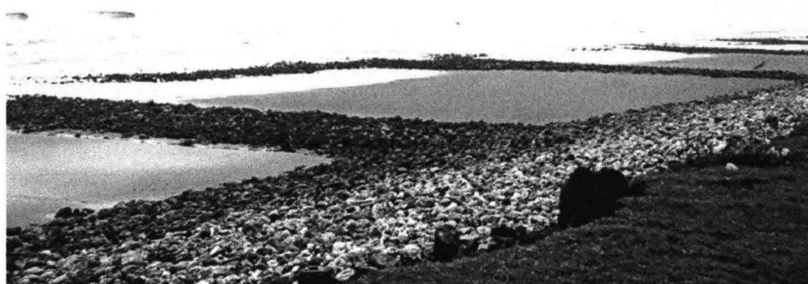
Fig. 3.6: Groynes with insufficient impact on the longshore sediment transport
