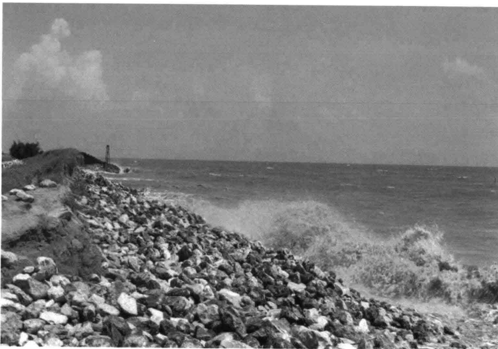
Fig 1.3: A damaged dike section
