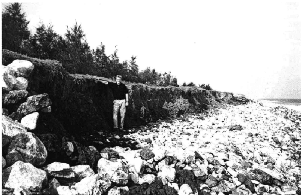
Fig. 2.9: Severely eroded dike with planted casuarina trees at Hai Hau beach.
