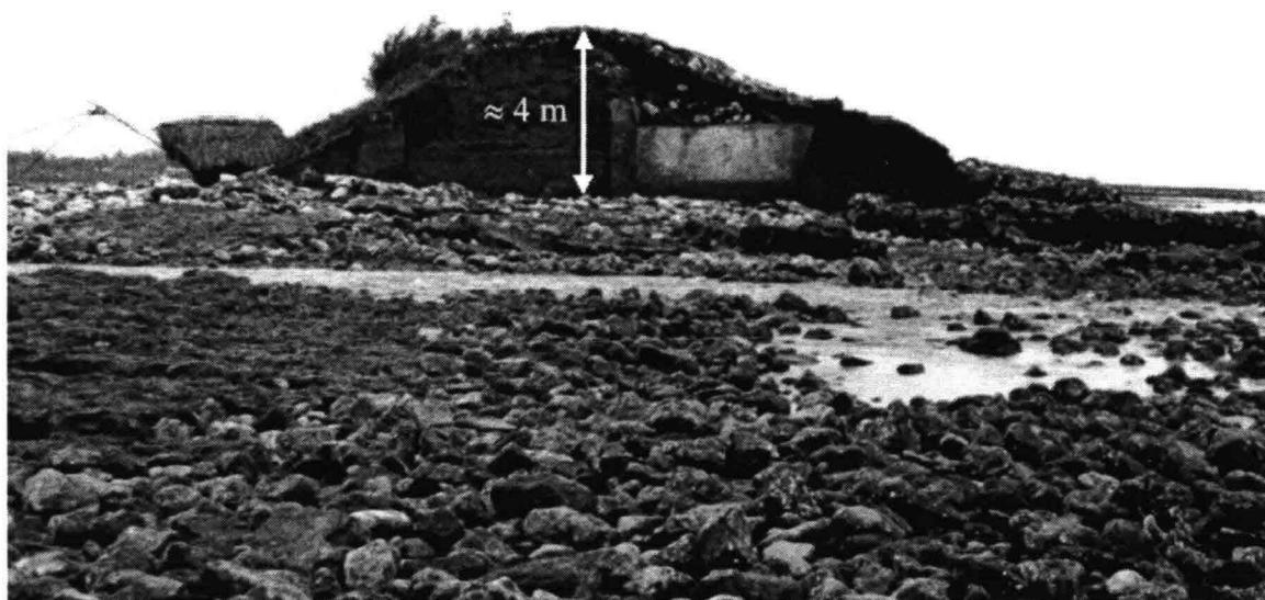
Fig.2.10: Characteristic cross-section of an eroded dike near Van Ly village
