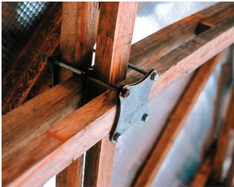
Figure 30 Nodal Connection of the Weald and Downland Gridshell [Cullinan Studio, n.d.]
