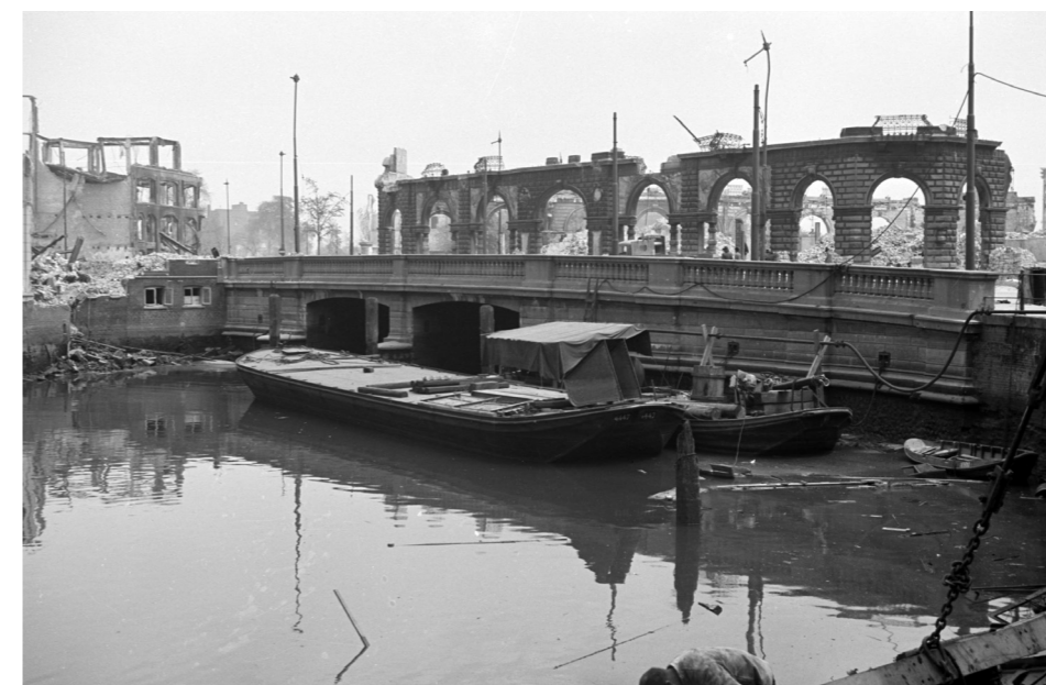
Figure 19. The Kolk hit by the bombing of 14 May 1940 with the facades Plan C in the background. Ships and pieces of debris lie in the water of the Kolk, 1980-5099, 1940, Gemeente Rotterdam (Stadsarchief). Accessed April 10, 2024, https://hdl.handle.net/21.12133/32D32062F25C4D-01BE8905A751E96D76 .
