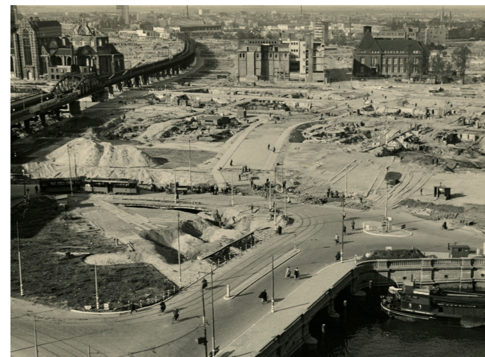
Figure 20. View from the Witte Huis of part of the Oudehaven and Oudehavenkade with surroundings, a bomb-damaged area, and further on the Municipal Library on Botersloot and Nieuwemarkt. On the left the railway viaduct and the Sint-Laurenskerk, IV-339-10, 1941, Gemeente Rotterdam (Stadsarchief). Accessed April 10, 2024, https://hdl.handle.net/21.12133/4466B1FC78EE-4924955B4A6BE07CF4D4 .
