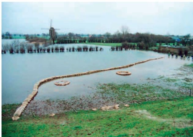
Figure 6 Sand boils during the high water of 1995
