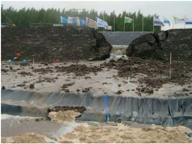
Figure 22 Breakthrough of the levee in experiment 1
