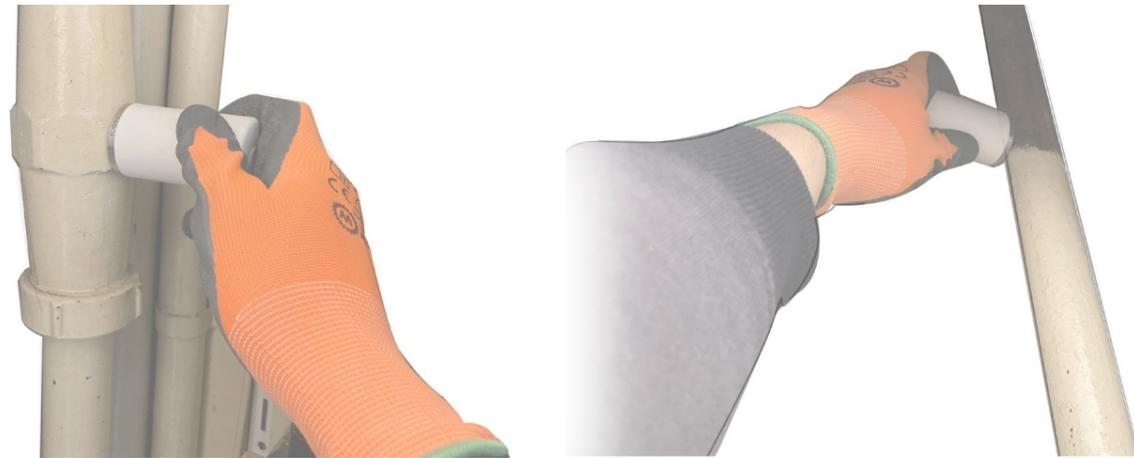
Figure 38: Edge Dynamics sensor node magnetically mounted
