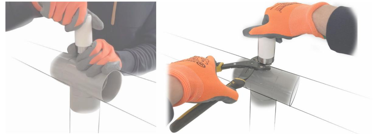
Figure 40: Edge Dynamics pressure sensor mounted, unscrewing by hand (left), unscrewing using tool right)
