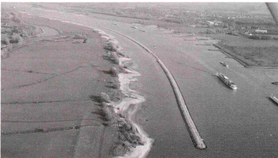
Figure 5. Longitudinal Training Wall (LTW) in the Waal branch of the Dutch Rhine River. (source: Rijkswaterstaat).
