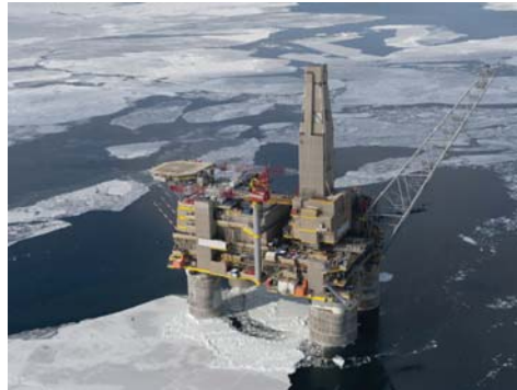
Figure 1.1: Lunskeye-A platform in level ice conditions in the Sea of Okhotsk, Russia (photo courtesy of Sakhalin Energy Investment Company Ltd.).
