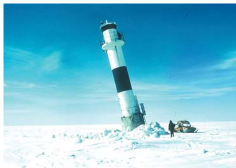
Figure 1.4: A Swedish lighthouse toppled by level ice (photo courtesy of Lennart Fransson).
