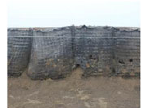
(b) Sand and soil filled wall
