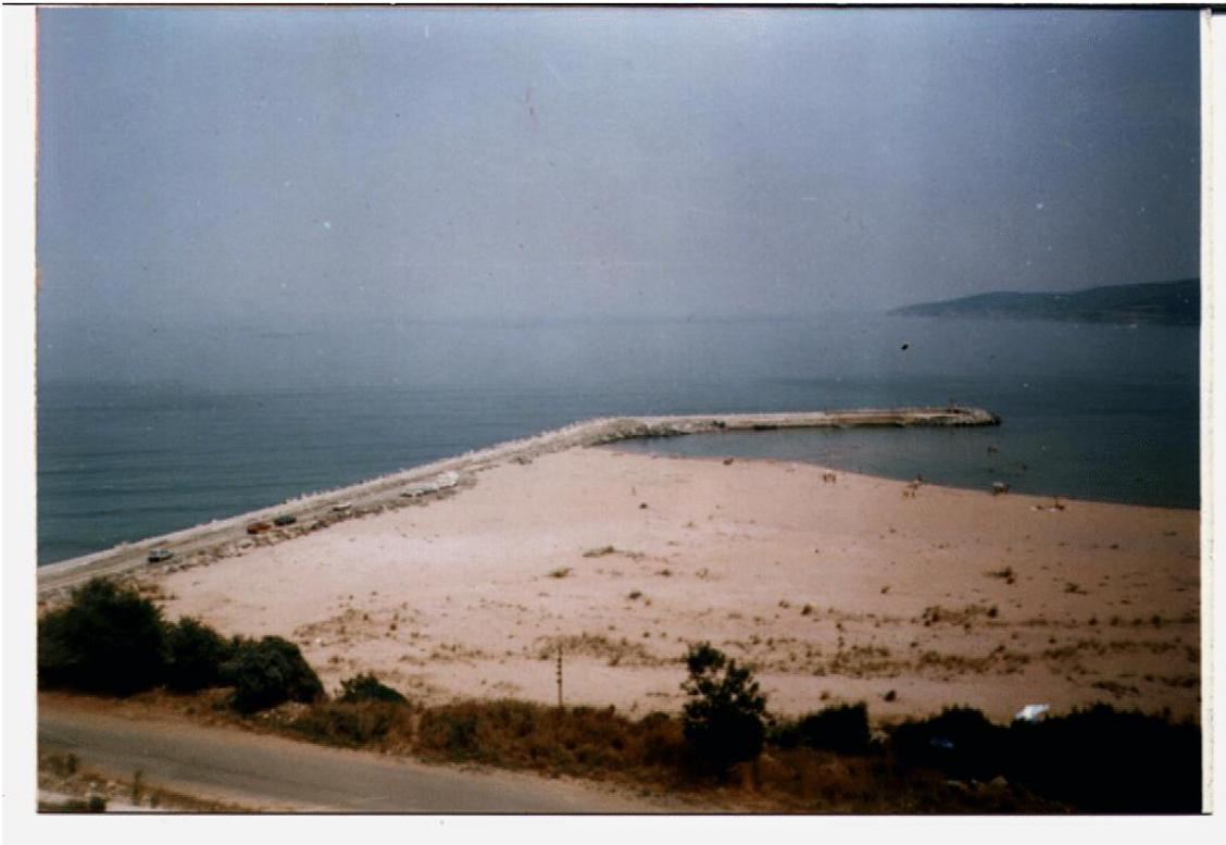
Figure 4: Sedimentation in the fishing harbour of Alepu
