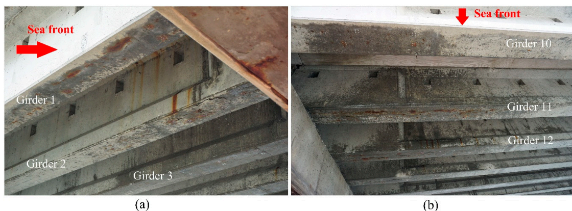
Figure 4. Corrosion-induced damage and humid areas in NIB girders: (a) in the first bridge span (1st to 3rd girders facing the sea) next to the middle support; (b) in the second bridge span (1st to 3rd girders facing the sea) next to the middle support.
