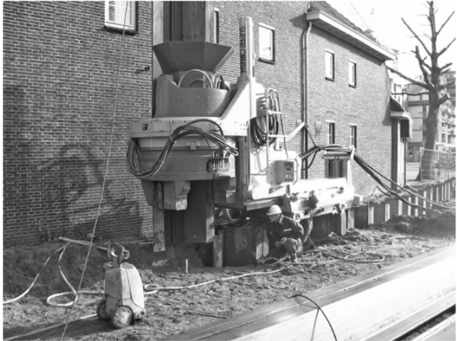
Hydraulic jacks that press piles into the ground_Giken Europe BV, London
