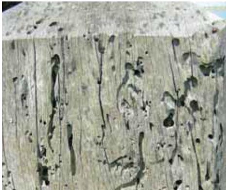
Figure 1 Results of marine borer attack
