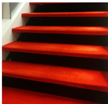
**Figure 4.5:** Staircase at the Faculty of Architecture in Delft, with no concrete vertical riser
