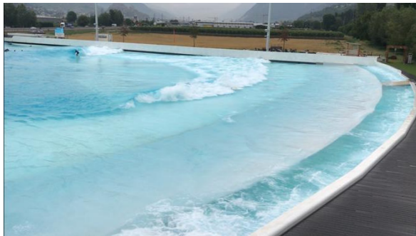
(e) Fifth time instant: the turbulent water in the gutter calmed down. The water level in the gutter is now elevated a little bit above the crest of the edge. The water from the gutter can run down the slope of the edge back into the wavepool.
