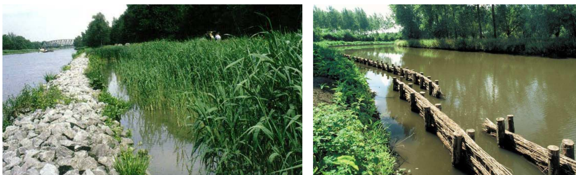
Figure 2.29: Left: detached breakwater with a wet strip. Right: fascine fences with wet strip (CUR, 1999).
