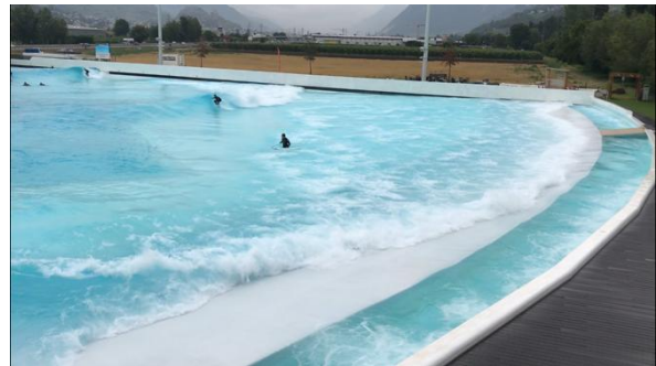
(f) Sixth time instant: the second wave is running up the slope of the edge. The water level in the gutter is still elevated up to crest level. Because of the elevated water level, less wave energy can be eliminated from the wavepool. It is difficult to see this in the screenshot.
