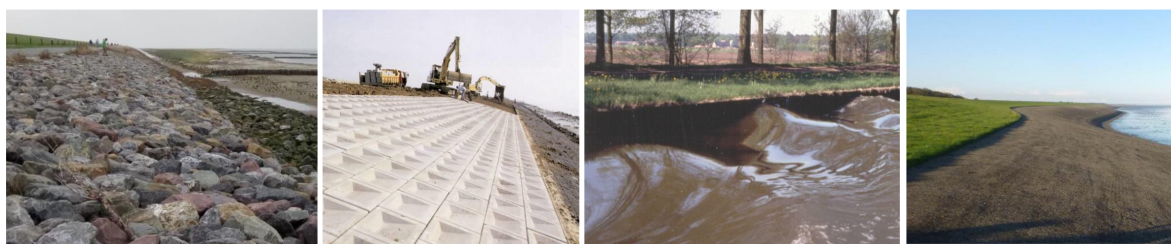
Figure 2.27: Types of hard bank protections. Left to right: Loose rock revetment, placed blocks revetment, vertical sheet pile walls, asphalt (Schiereck, 2017).
