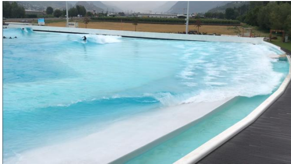
(c) Third time instant: the broken wave overtops the crest of the edge. Along the edge, water is deposited in the gutter by means of a water jet. The water jet has not reached the vertical wall behind the gutter yet. The water level in the gutter is not affected yet by the wave run-up.
