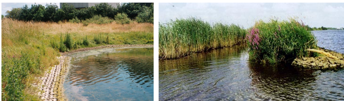
Figure 2.28: Grow-through protections or reinforced vegetation (en Waterbouwkunde, 1993).
