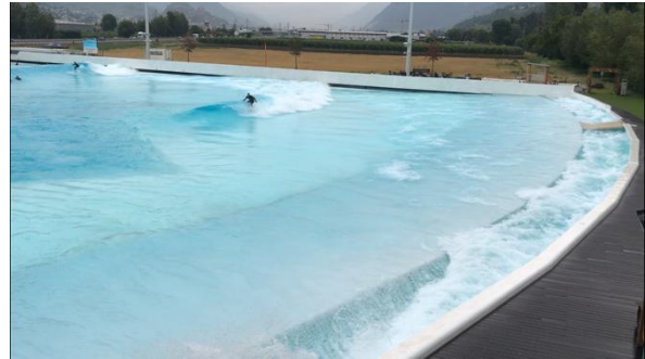
(d) Fourth time instant: the back of the broken wave runs down the slope of the edge back into the wavepool. The water jet is reflected back into the gutter by the vertical wall behind the gutter. This causes the water in the gutter to be very turbulent.
