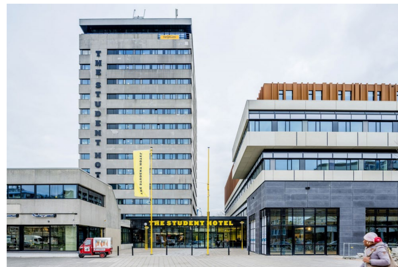
Image 3.20 Former offices of Het parool and Trouw are turned into student housing (duurzaamgebouwd.nl)
