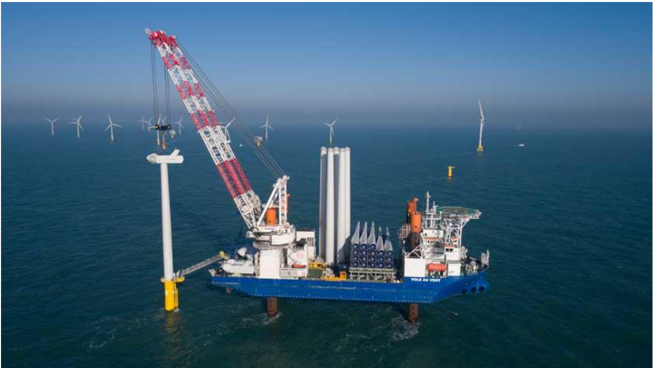
Figure 11: Wind turbine installation using a jack-up vessel (source: jandenul.com)
