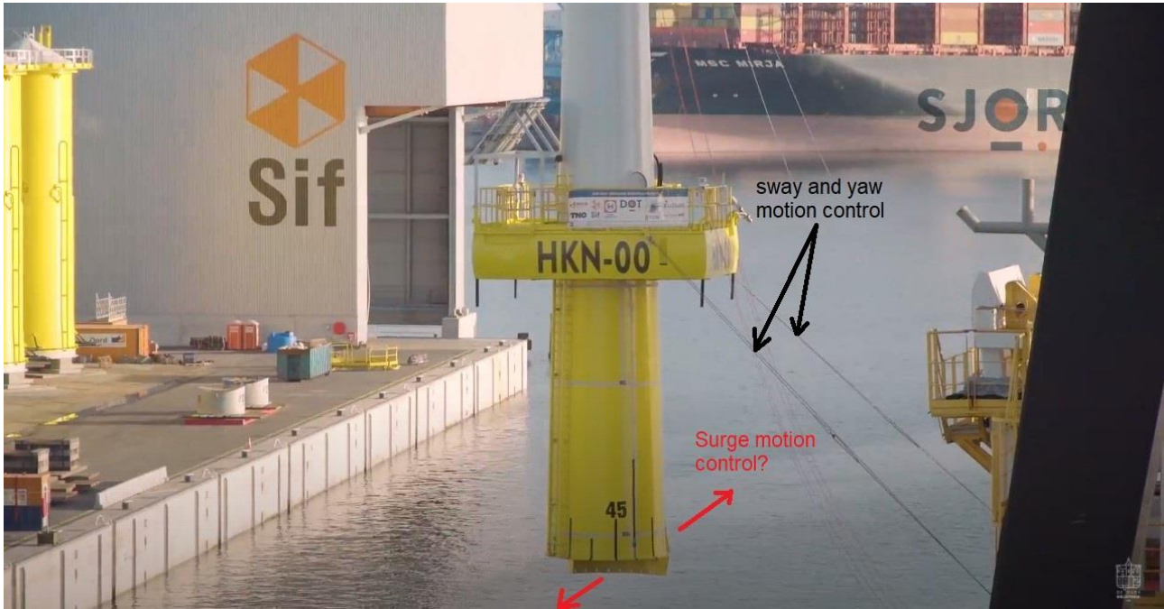
Figure 60: Installation of a WTG tower using a vertical asymmetric catcher. Tugger lines control the sway motions, suggesting that the WTG tower motions are primarily in the surge direction (source: https://www.youtube.com/watch?v=4f3qkd_oaCs )
