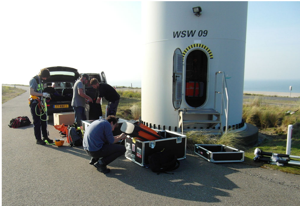
Figure 36: Onno (TotalWind), Teus (Vattenfall), Erik and Chris (Oldbaum Services) preparing equipment for installation
