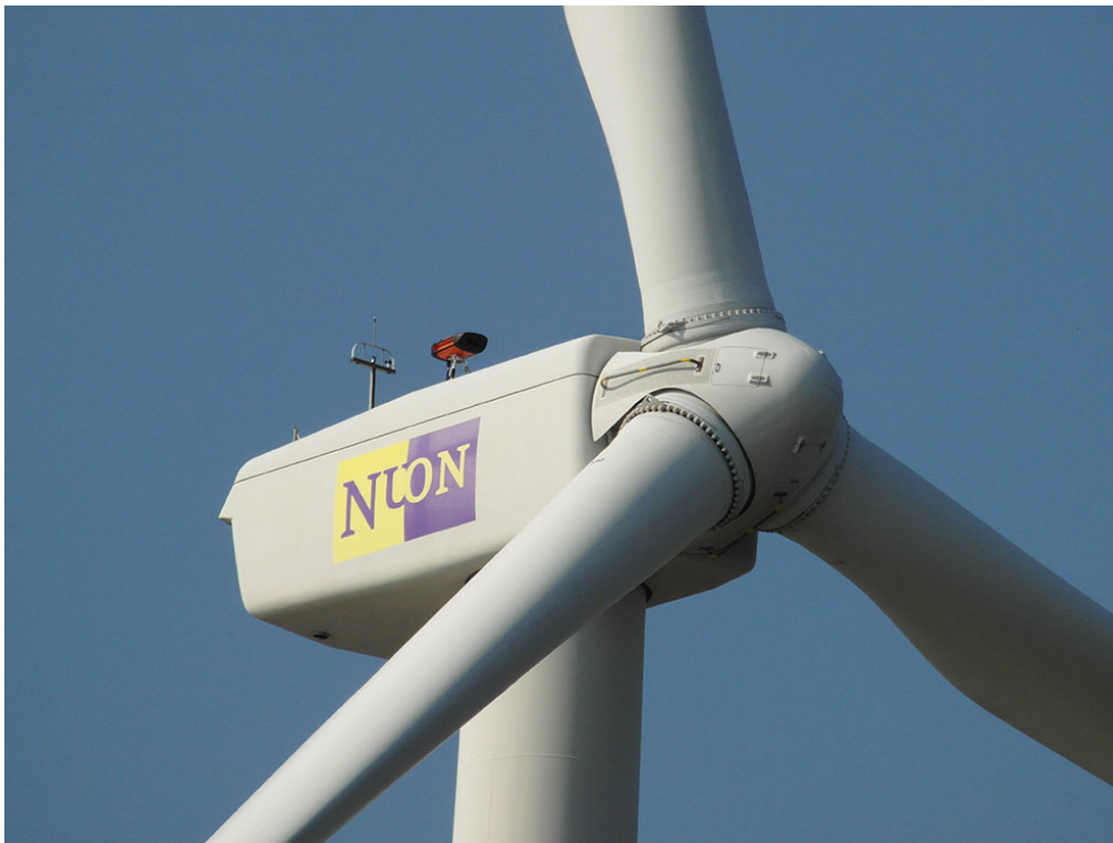
Figure 39: Wind Iris successfully installed on Wind Turbine 9 of Slufterdam West
