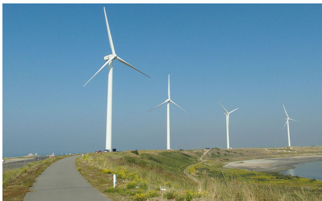
Figure 5: Left to right: Wind Turbine 9, 8, 7 and 6 of Slufterdam West
