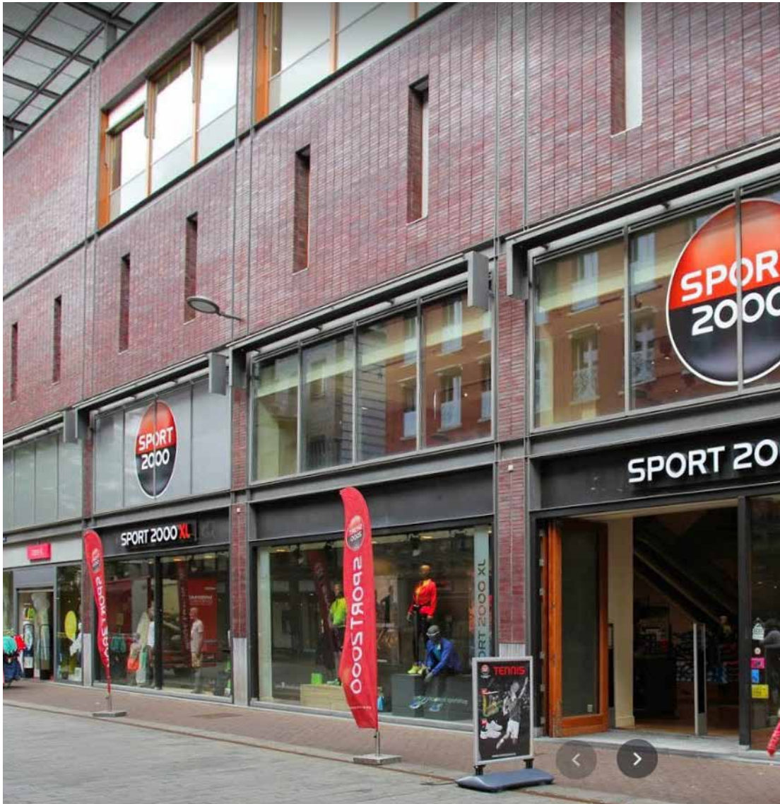
10. PHOTO OF THE CURRENT SITUATION OF THE STATENPLAATS FACADE
