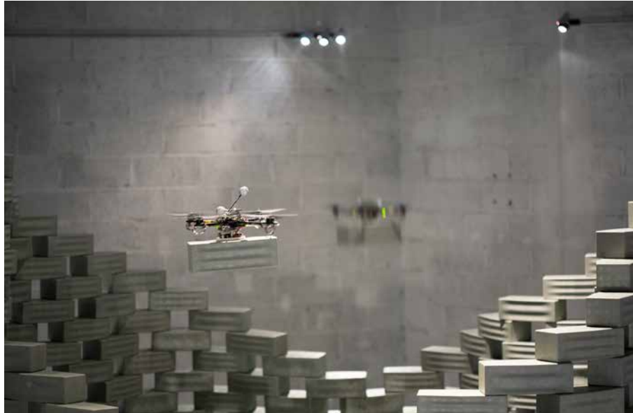
FIGURE 5.5 Flight Assembled Architecture by Gramazio & Kohler (source: ETHZ, Gramazio & Kohler Research and Institute for Dynamic Systems and Control, http://www.idsc.ethz.ch/research-dandrea/research-projects/archive/flying-machine-enabled-construction.html )
