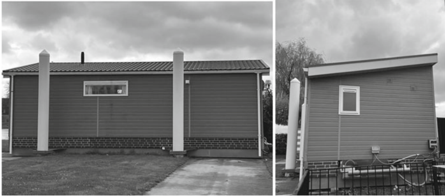
Fig. 4 Chalet originally built as a “stacaravan” in 2013 transformed into an amphibious building in 2022 using an aluminium buoyant foundation (images taken by author)
