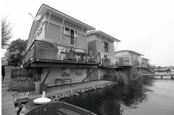
Fig. 1 Amphibious homes in Maasbommel in July 2016 seen from the jetty. Concrete buoyant base visible under the terrace (image taken by author)
