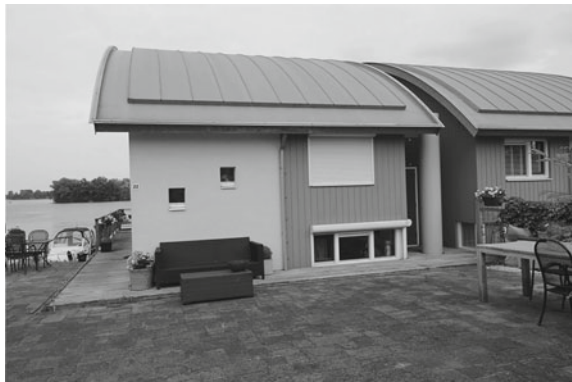
Fig. 2 Amphibious homes in Maasbommel in July 2016 seen from the road. Steel dolphin pile visible between houses. Maas River in the back (image taken by author)
