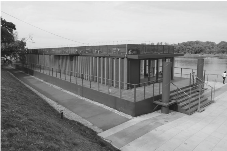
Fig. 9 The first pavilion finished in September 2016. Semi-wild Vistula River is visible in the back (image taken by author)
