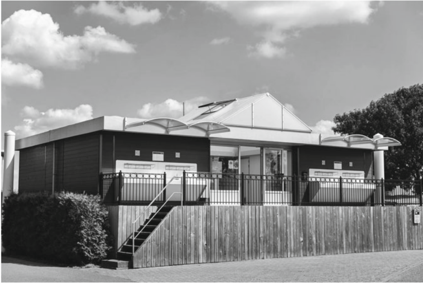
Fig. 3 Amenity building with concrete buoyant foundation ( source Resort Marina Oolderhuske)
