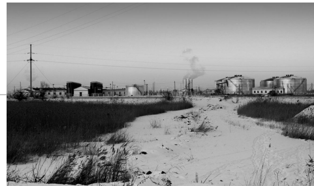
Oil transferring station
