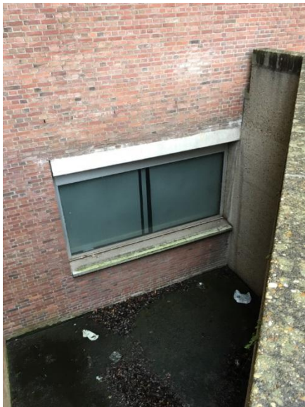
Fig. 9: The window well and the window with closed louvers.
