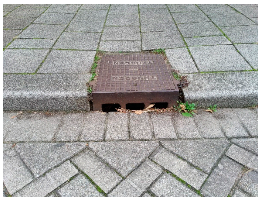
Figure 1. Roadside gully pot.
