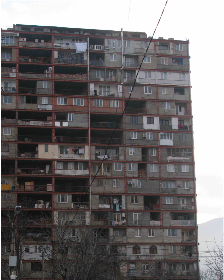
kamikaze loggias reinforced by municipality of Tbilisi
