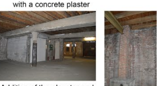
8. Addition of a brickwork fireplace
