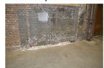
11. Expansion of the concrete floor up to the facade
