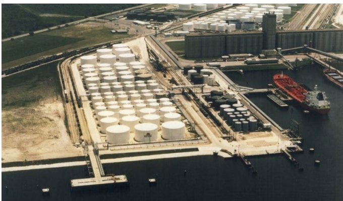
2.14 Deer Park in Houston, 1976, liquid storage facility.
