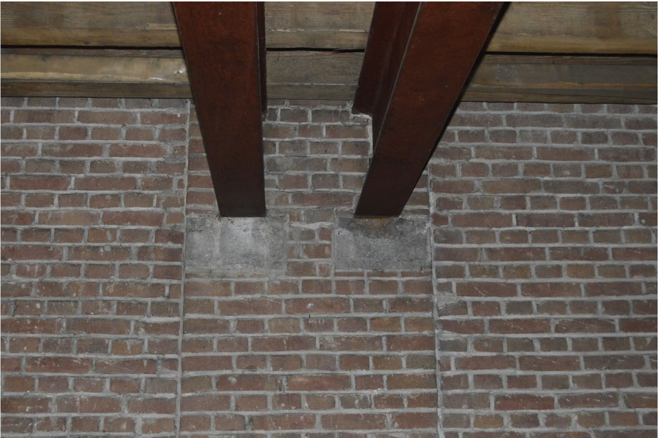
4.01 Picture of the iron beams imposed within the brickwork on top of two larger natural stones.
