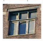
10. Replaced window on the 5th floor
