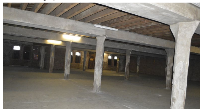
3.35 Picture showing the oversight of space, taken on the first floor
