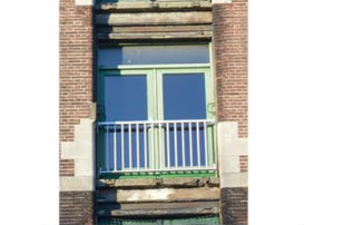
3. Filling of the 3rd floor door openings with glass doors and a metal railing
