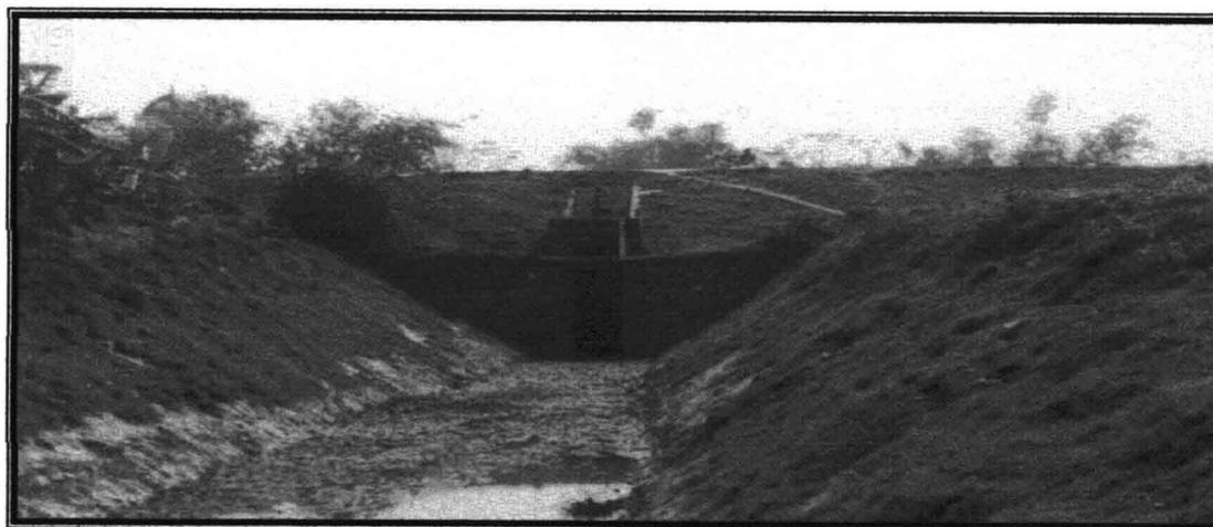
Figure 3.7 A typical conduit under the right Duong River dike
