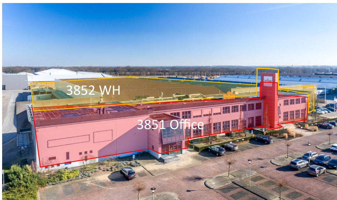
Figure 23 - K3851 office and K3852 Warehouse (From PERE firm)
