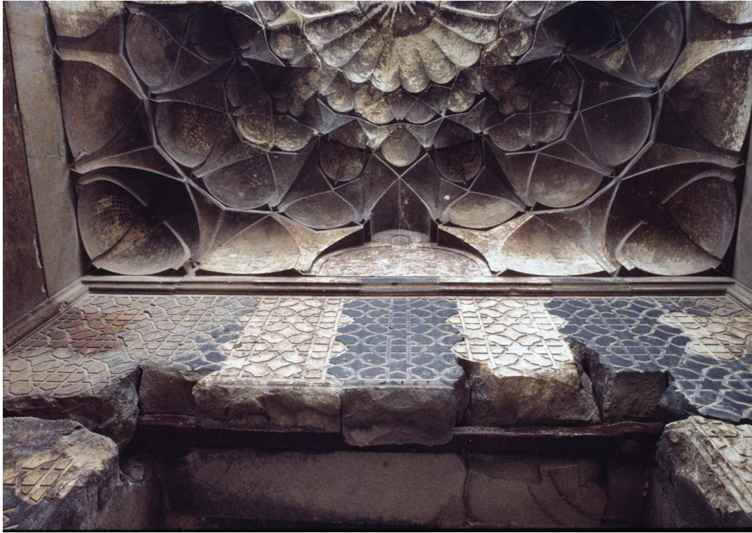
Figure 27: Ayyubid Palace entrance portal: view of muqarnas hood from below with the typical Ayyubid masonry work of striped limestone decorated with geometric patterns. From Archnet , by Tabbaa, 1990
