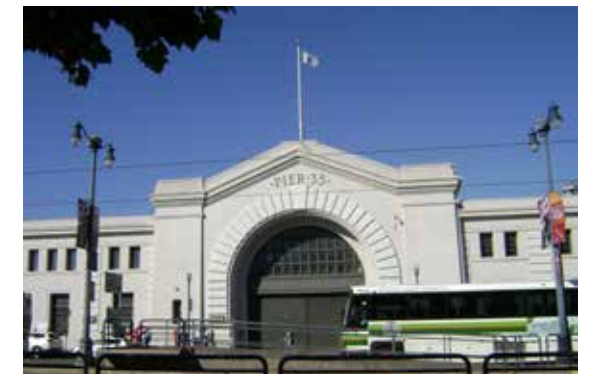
Pier 35 Bulkhead Building
