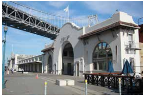
Pier 28 Bulkhead Building
