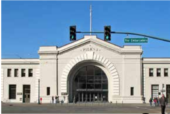
Pier 1 Bulkhead Building
