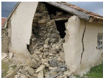
Figure 2.2: Examples of failure mechanisms in masonry structures: (a) classification [34], (b) diagonal shear sliding [35], (c) diagonal crack, (d) rocking failure with flexural cracks and toe crushing [36], (e) vertical splitting and crushing of masonry bricks [37], (f) crumbling and out-of-plane failure [38].
