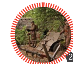
Fort Mistrzejowice 1897 - Kraków Stronghold Line (devastated)
