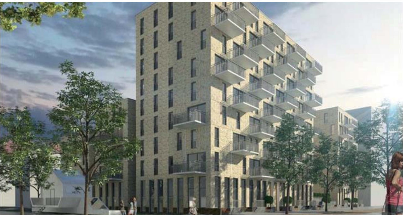
Figure 1 - Exterior Coubertin Zeeburg
