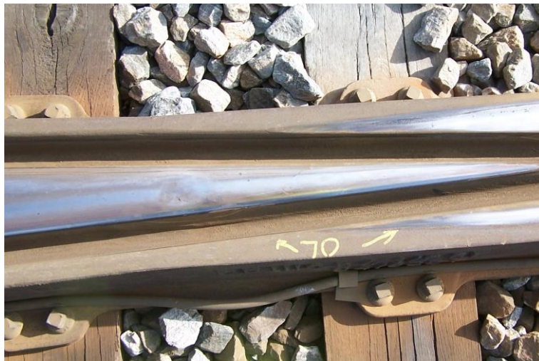
Figure 2.1. RCF damage at railway crossing
