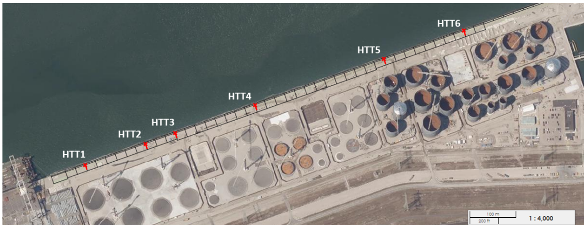
Figure B.8: Satellite photo of HTT quay wall
