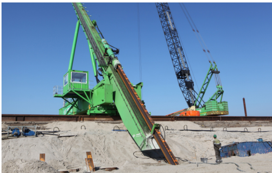
Figure 2.3: Installation of MV pile (personally taken photograph: Putteman, J.).
