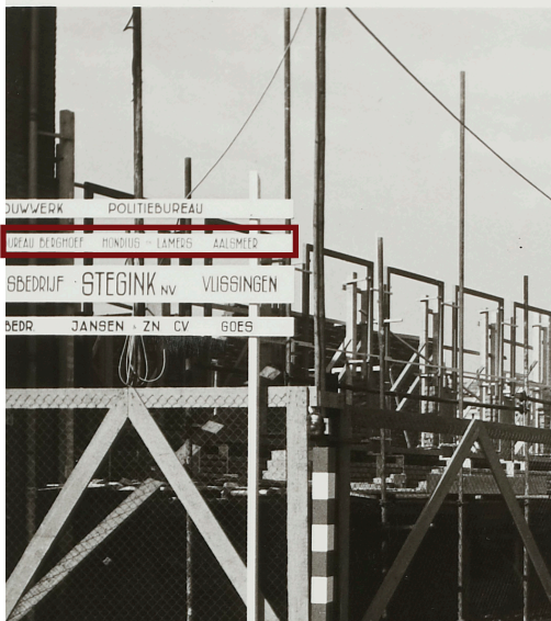
Police station under construction. Zeeuws Archief
